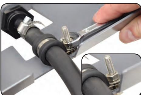
7. Use washer on both sides of base. Insert 10mm bolt from bottom side and tighten nut to clamp down tubing and provide strain relief.
